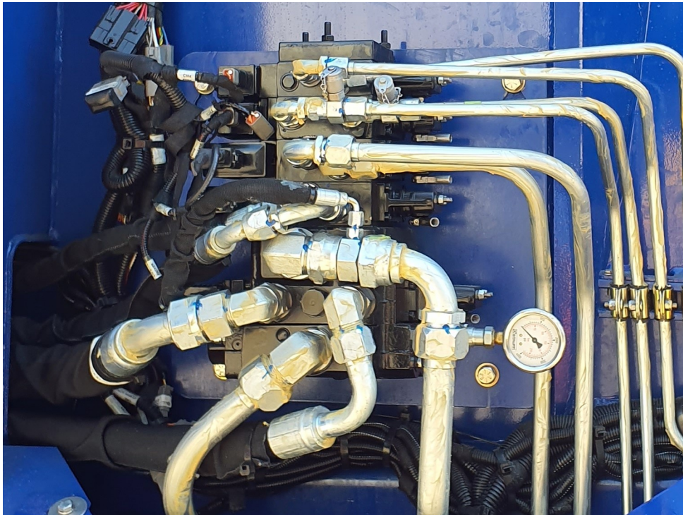
Figure 7-20 Main valve (protective cover removed)
